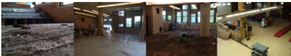
Figure 3. Learning environments prior to renovation and construction
