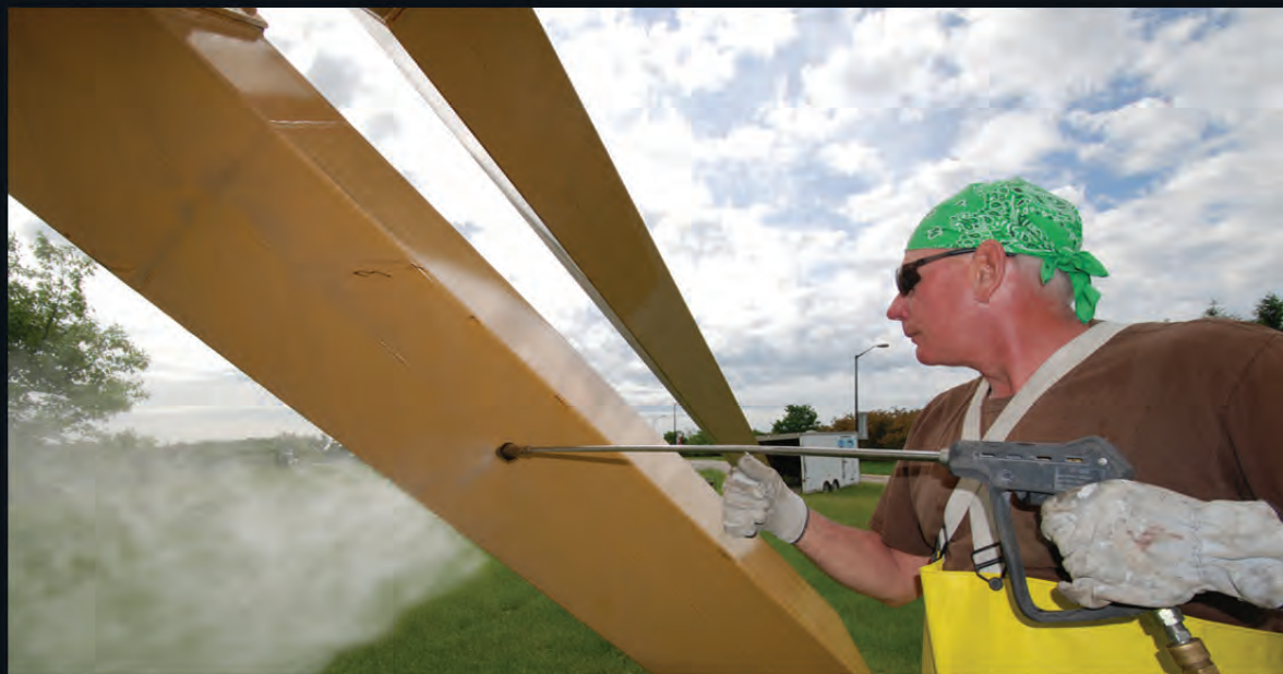
Above: Madison Coatings' Gary Goins conducted the work on Illinois Landscape No. 5 . Goins began by powerwashing the entire surface of the sculpture, removing the chalky residue of paint present since its last painting in 1997. Note the pale buttercream hue.
