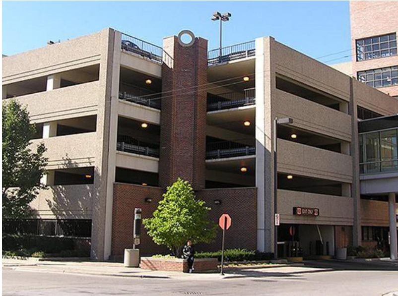
Wood St. Garage (Parking Office)
